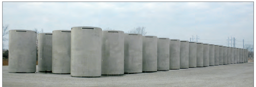
Top photo: The last MAGNASTOR system is transported to the ISFSI pad at Zion. Bottom Photo: NAC MAGNASTOR spent fuel casks on the Zion ISFSI pad.
