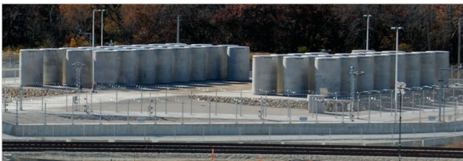
Top right photo: Cask temperatures are continuously monitored at the ISFSI. Bottom photo: NAC MAGNASTOR spent fuel casks on the Zion ISFSI pad.
