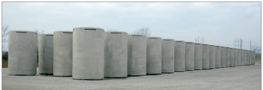
Top photo: The last MAGNASTOR system is transported to the ISFSI pad at Zion. Bottom Photo: NAC MAGNASTOR spent fuel casks on the Zion ISFSI pad.
