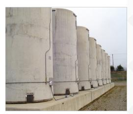
**Top photo:** NAC MAGNASTOR spent fuel casks on the Zion ISFSI pad. **Bottom Photo:** Cask temperatures are
